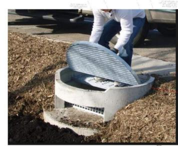
USE AN INLET STRUCTURE SIMILAR TO INLET SHOWN IN PICTURE
