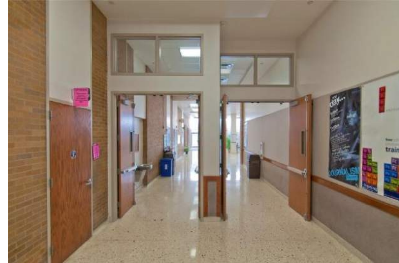
Double egress fire doors in open position
