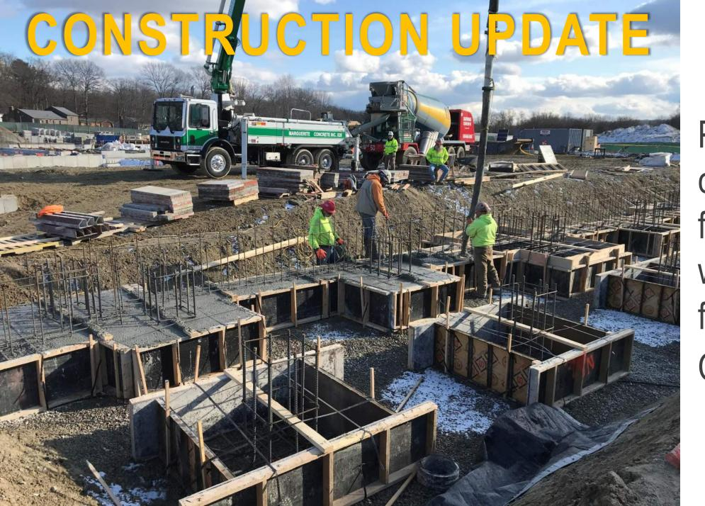
**Placing** concrete footings, West wall & canopy foundations C Wing
