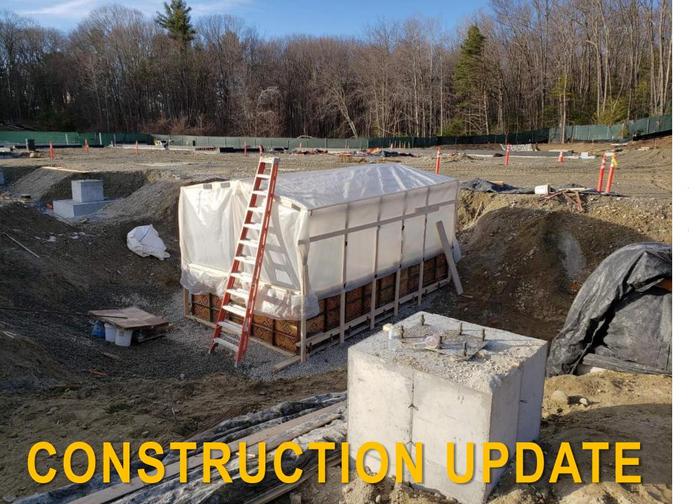
Weather/ heating tenting for curing concrete, elevator pit foundation
