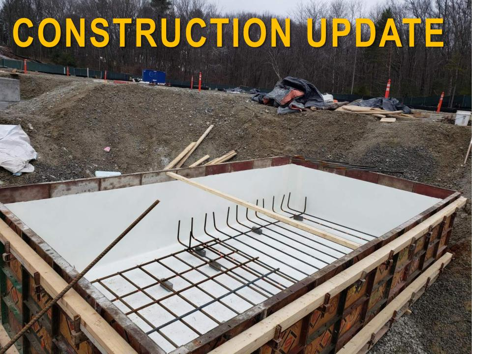
Blind-side waterproofing, elevator pit foundation
