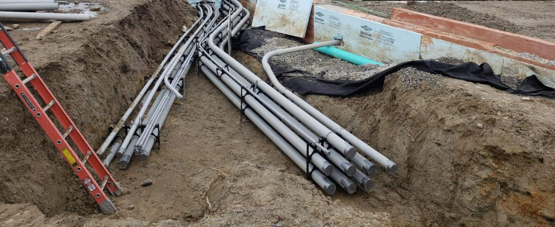
Electrical secondary conduits heading toward the main transformer
