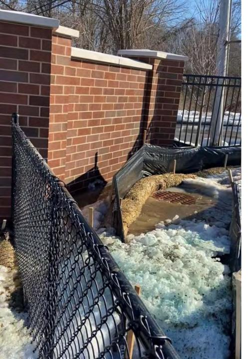
Added grate inlet to top of manhole structure. May add another one – Civil Engineer is studying.
