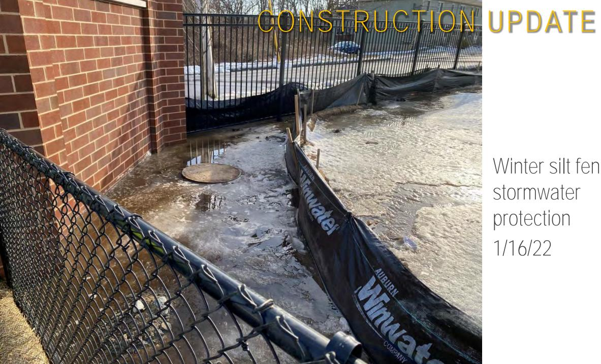
Winter silt fencing: stormwater protection 1/16/22
