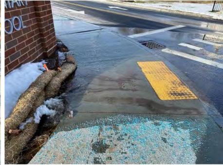
Winter silt fencing and straw wattles: stormwater protection 1/16/22
