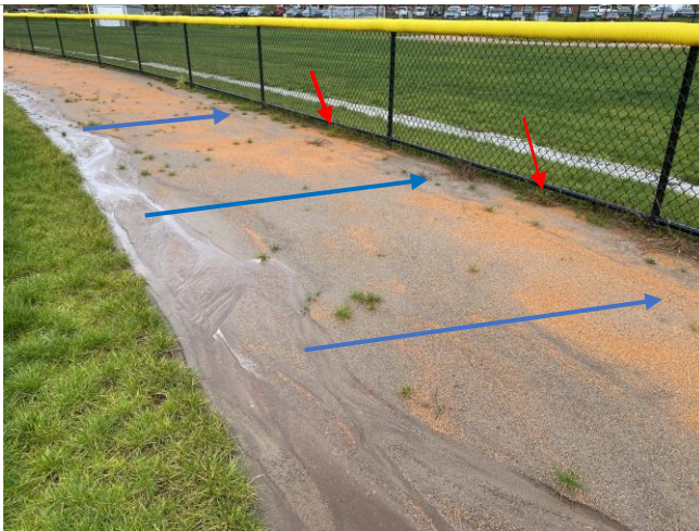
Photo 1 – Baseball warning track – slope (blue) and reduce lip (red)
