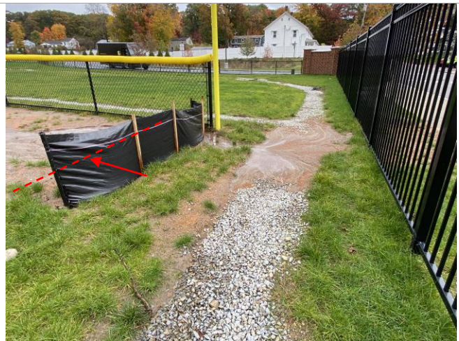
Photo 2 – Eroded area to be repaired – move silt fence as shown
