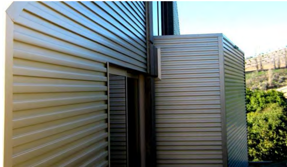
Panel Material: Corrugated metal siding
