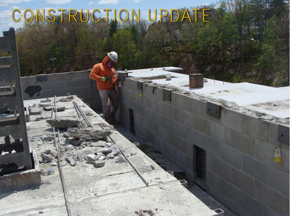
5/12/20 – Stair #3 Masonry progress – topped out and adding outrigger supports
