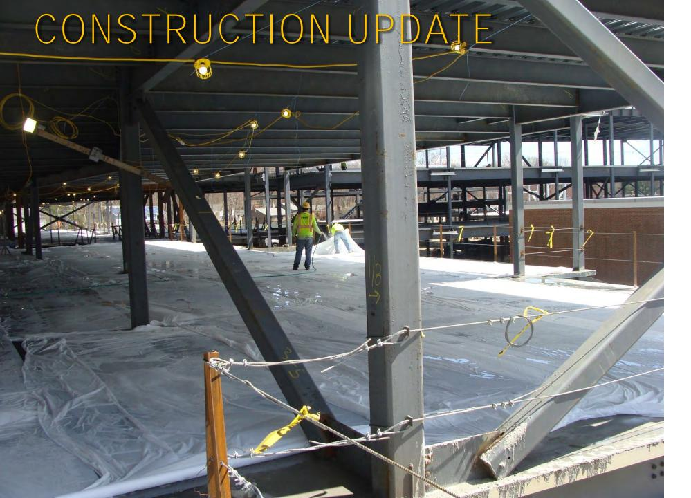
4/7/20 – Slabon-deck wet curing underway: A-Wing, Level 2
