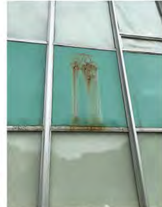
Leaking, rusting, inefficient window systems
