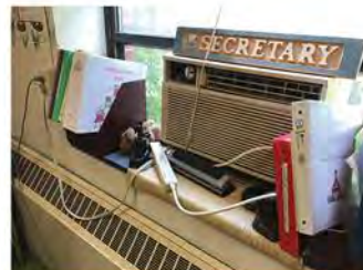
Insufficient electrical outlets
