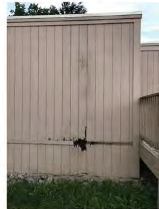
Modular cladding rotting
