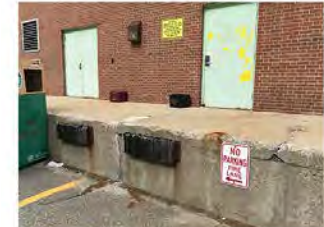
Cracking, disintegrating concrete
