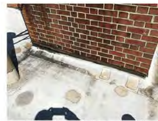
Patched leaking roof
