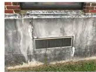
Cracks in concrete foundation
