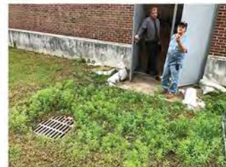
Poor site drainage, water runs into building
